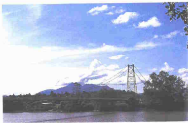
13. The Satok Suspension Bridge was built in 1926 and formed a link between the north and south banks of the Sarawak River. (Darrell Tsen)
